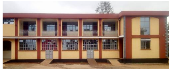
Completed building of the Fire & Rescue Training Centre in Kiambu. The Centre has a capacity to train around 40 persons.
